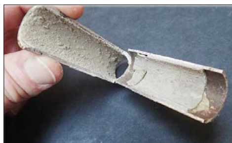
Figure 2: Calcium carbonate scale in a heat exchanger tube.
